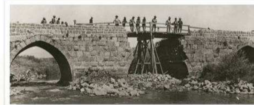
Above, top: The bridge had a long history of war even before World War I: here the bridge is depicted in 1799, with British forces occupying the mountain in the distance during Napoleon's advance through the region
